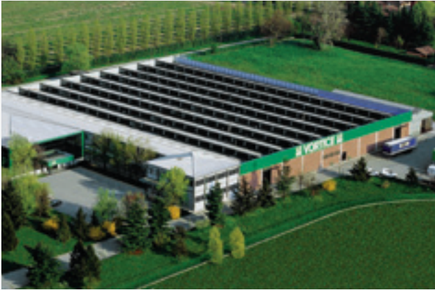
Our current Vortice Headquarters have been located in Tribiano (Milan) since 1972.
